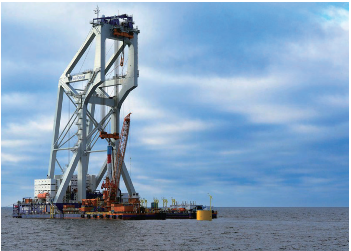
Baltic Power海上风电场首台风机基础 来源：Baltic Power, balticpower.pl
