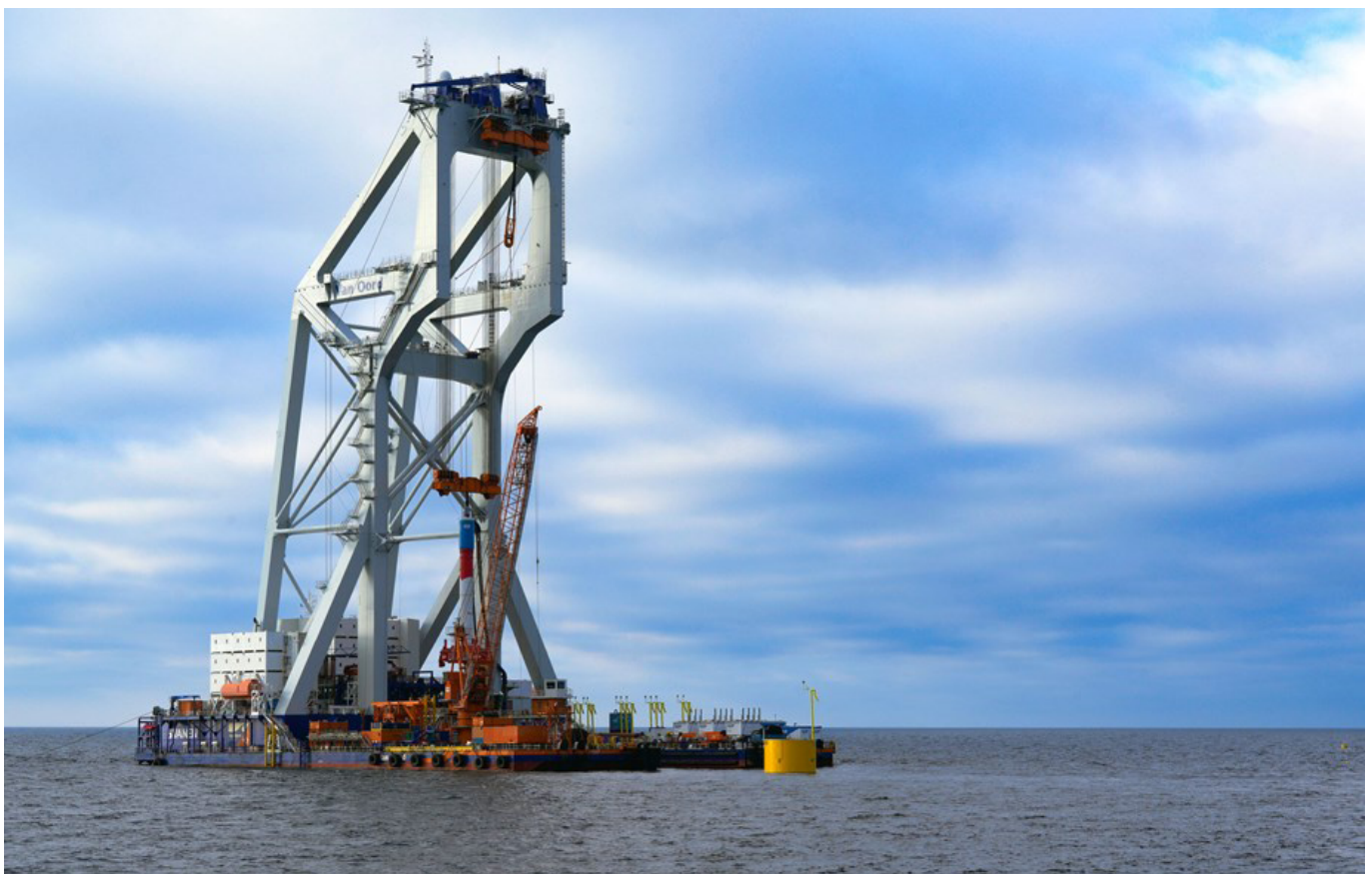
The first foundation of the Baltic Power wind farm
