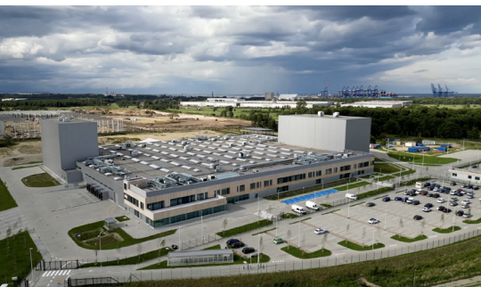
Northvolt Dwa ESS, the largest energy storage systems manufacturing facility, which was acquired by Lyten.
